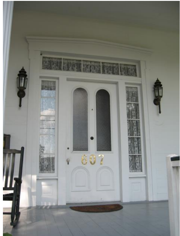
Architectural details such as this two-arch-light door and multi-light sidelights and transom are highlights of the dwelling at 607 2nd Street. Known as the Oliver-Todd House, it was built in 1854 for Jules Oliver.
