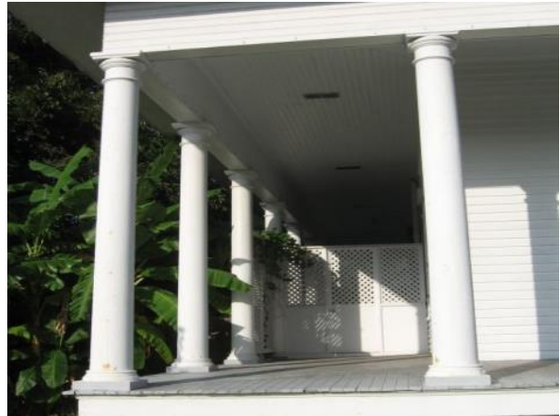
Retaining historic material on porches like the Tuscan columns on at 817 Main Street enables buildings to retain integrity.
