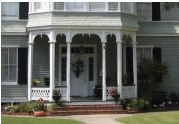
The Queen Anne porch trim at 307 Main Street is an important visual component of the house.
