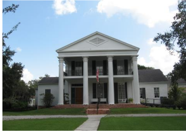
The Palfrey House at 200 Main Street was built ca. 1851 by Gov. Joshua Baker for his daughter Frances Baker Palfrey. Its imposing portico defines its Greek Revival character and should not be altered in any way.
