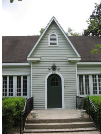
The arched entrance and projecting entry bay with steep gable roof at 601 Adams Street support the house's Tudor Revival character.
