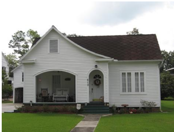
The house at 615 Adams Street includes many Tudor Revival features; the multiple steep gable roof and arched entrances are prime examples. Multi-light casement windows are also common to the style,.
