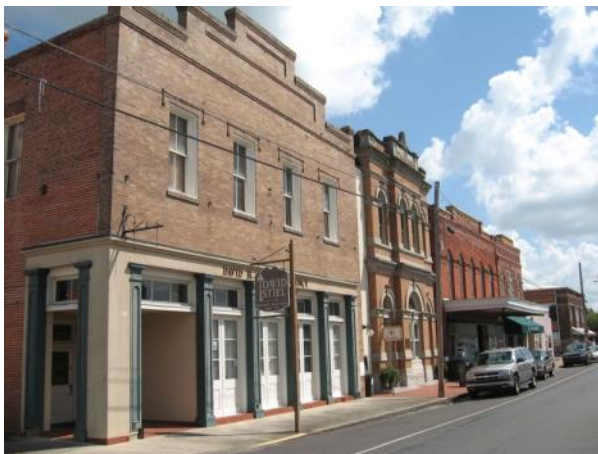
Flat roofs are a hallmark of historic commercial buildings. (600 block Main Street)
