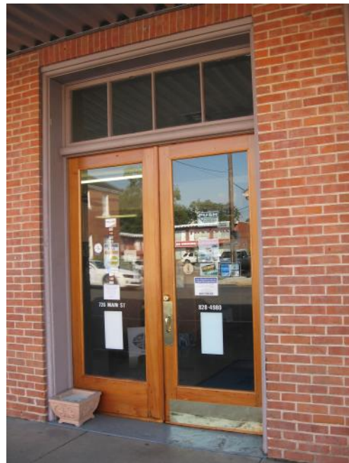
Single-light glass and wood doors are appropriate designs when rebuilding traditional storefronts (726 Main Street).
