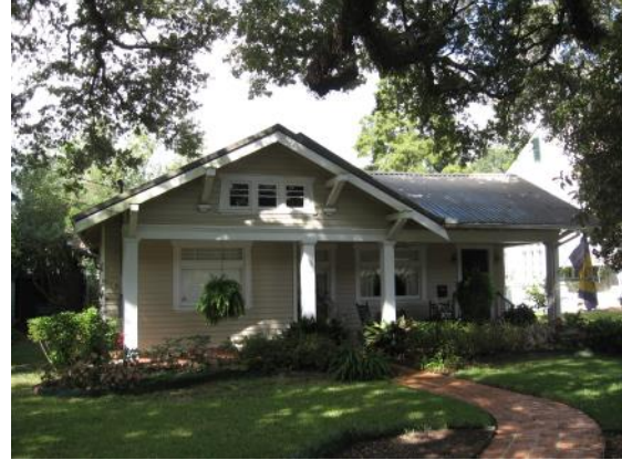
Stylistic elements at 905 2nd Street include multi-gabled rooflines, brackets under the eaves, and a wide porch.
