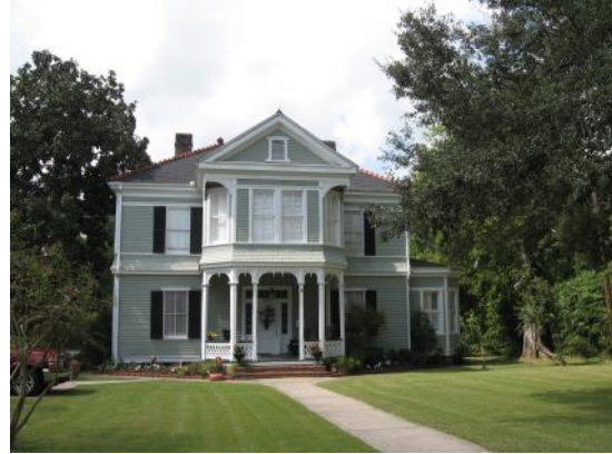
The Frere-O'Neill House at 307 Main Street shows influences of the Queen Anne style including various surface planes, wood shingle exterior trim, cresting on the rooflines, and milled porch trim and posts. The property was once owned by the late Charles Austin O'Neill, Chief Justice of the Supreme Court.
