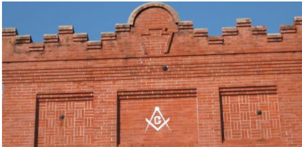
The detailed corbelling of the cornice at 709 Main Street contributes to the building's historic character.
