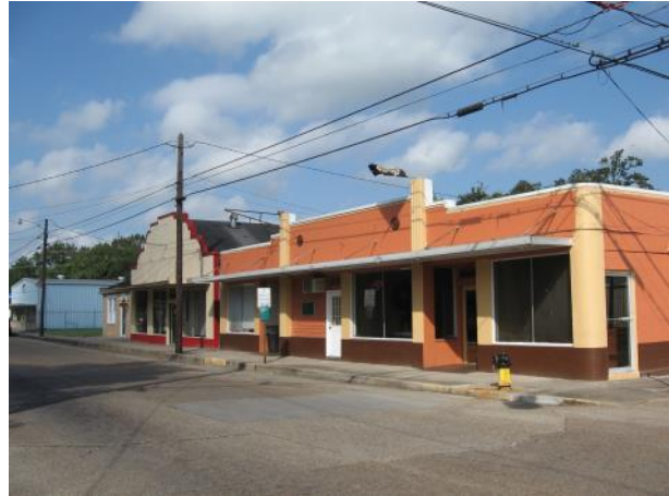
These early-20th century commercial buildings retain the typical storefront arrangements, covered by awnings and have modest decorative features, such as square pilasters and simple parapets.
