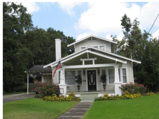
At 510 Adams Street is an example of what is called an airplane bungalow, with a multi-gabled roof and monitor atop the main roof.
