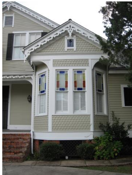
This bay window at 309 Adams Street exemplifies the variety of architectural detailing in the historic district and displays hexagonal wood shingles, eave vergeboard and windows with border glass in the upper sash.
