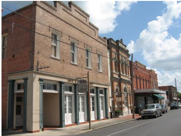
The buildings in the 600 block of Main Street show the rectangular plans, flat roofs, lower storefronts, sash upper windows, brick construction, and cornices so common to commercial buildings of the late 1800s and early 1900s.
