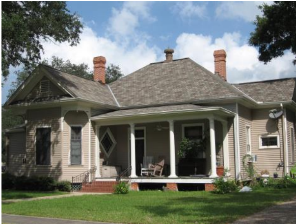
The interior brick chimneys at 614 Adams Street emphasize the asymmetrical floor plan of this folk Victorian dwelling.
