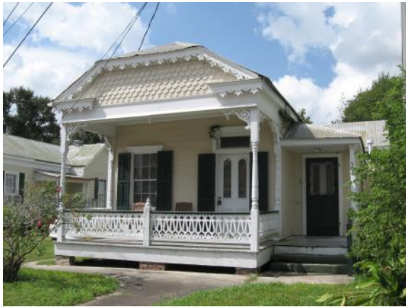
Original architectural features should be preserved and maintained. Replacement of original features should be with materials that match the original. (504 1st Street)
