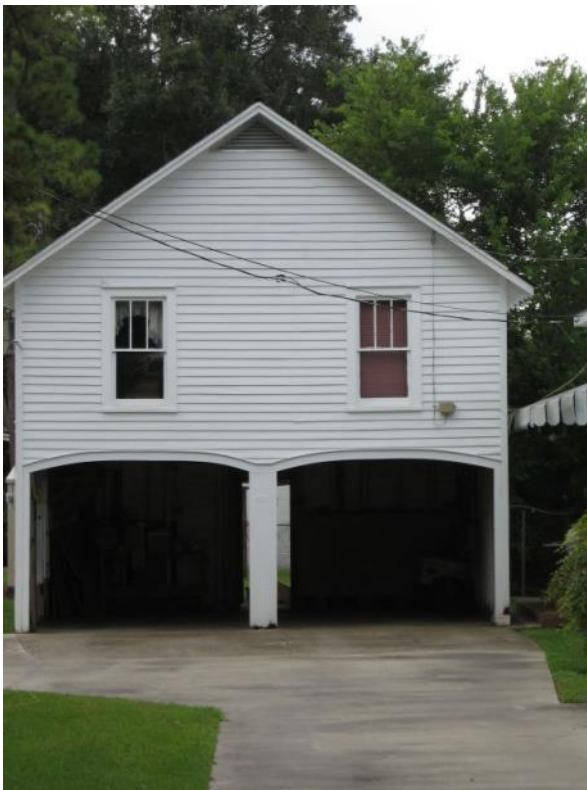
Outbuildings, like this garage at 615 Adams Street, were common in the early 20th century.
