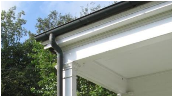
The gutter at 619 2nd Street uses an appropriate half-round design.
