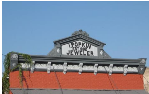
Metal cornices like the one on 615 Main Street were often used on commercial buildings from the late 1800s.
