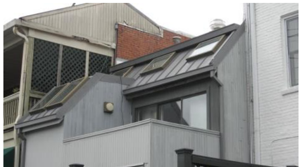
These skylights are appropriately placed.
