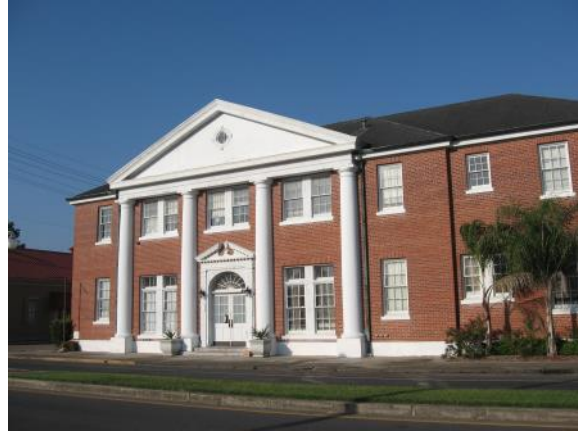
This building at 801 Main Street, constructed in 1938, has a large pediment, symmetrical façade, six-over-six sash windows, and classical columns, all elements of the Neo-Classical style.
