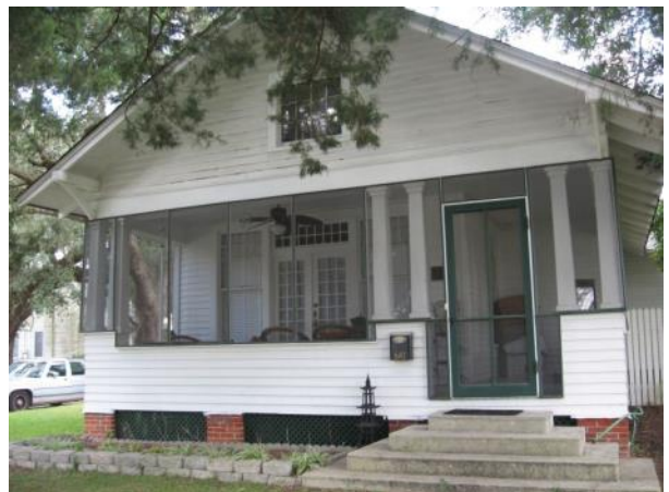
Shown at 610 1st Street is a model for enclosing a porch with minimal alteration or obstruction to its structural or decorative elements.
