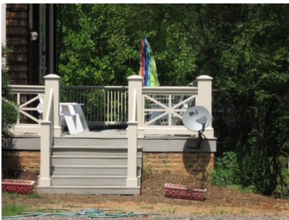
Satellite dishes should be mounted at rear elevations where they are not readily visible from the street.
