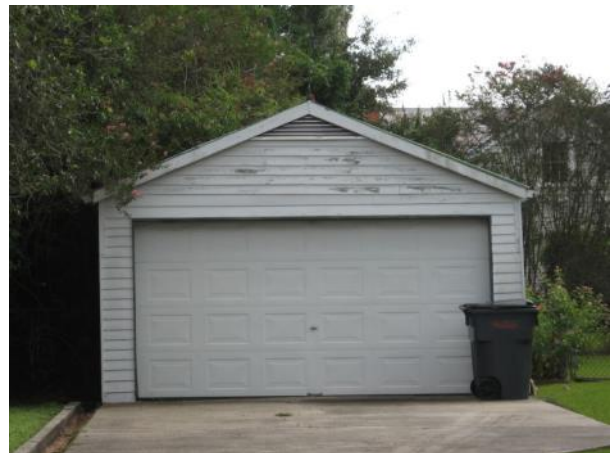
This garage at 914 2nd Street has a replacement door retrofitted to the opening.
