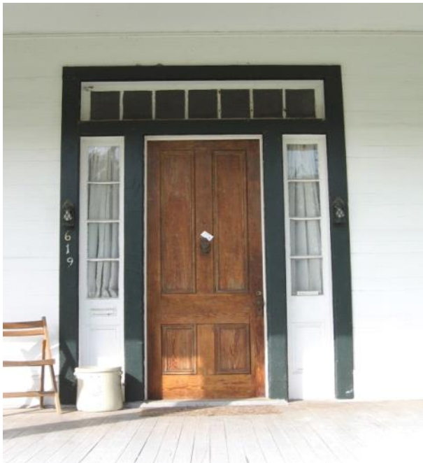
Six-panel wood doors, like this one at 619 2nd Street, are appropriate models for many Colonial Revival and Minimal Traditional dwellings, should replacement doors be necessary.
