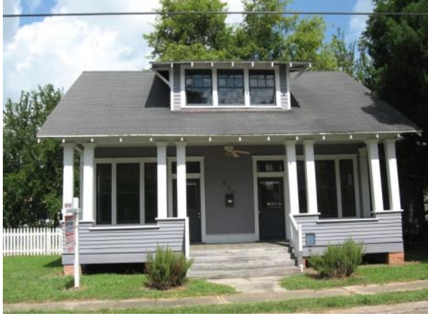
This dwelling's two entrances, with matching doors and transoms, should be preserved.
