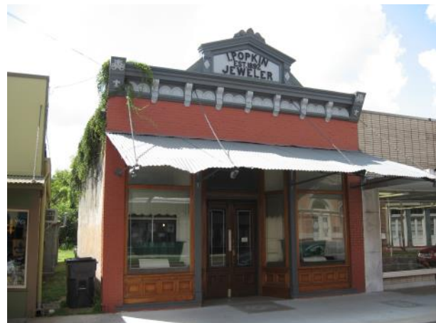
The building at 615 Main Street features typical elements of a one-part commercial building, including display windows on the first level, awnings over the windows, and decorative elements at the cornice.
