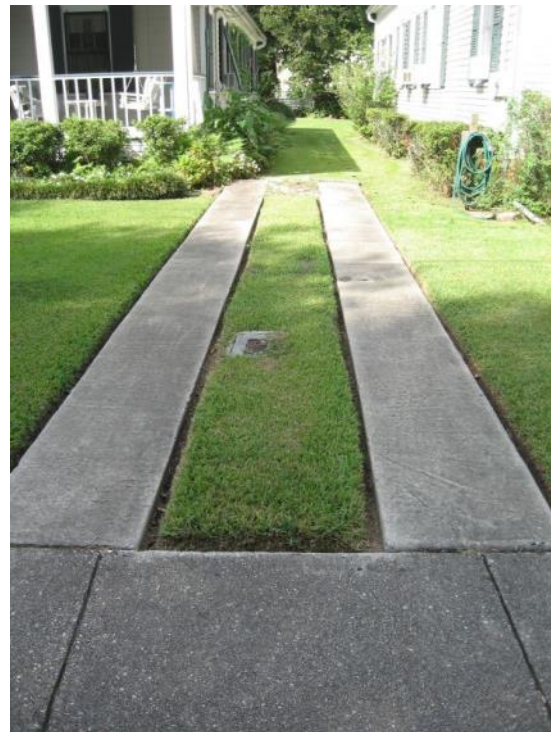
Concrete ribbons, like at 805 2nd Street, are common historical designs for driveways in urban neighborhoods.
