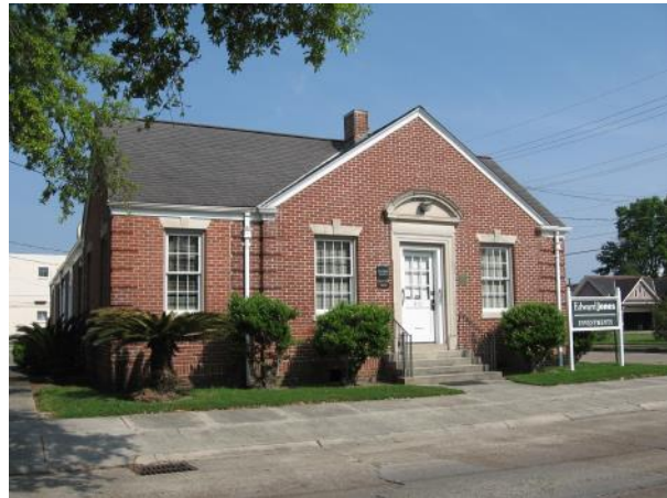
This building at 800 1st Street is constructed in the Colonial Revival style, with features such as a Classical entrance, brick quoins at the corners, and six-over-six and eight-over-eight double sash windows.
