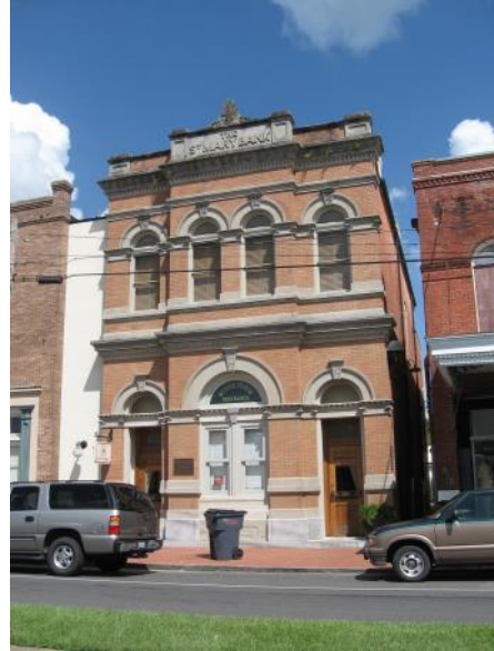
The building at 614 Main Street shows the influence of the Richardson Romanesque style, with its heavy arches, while retaining common commercial features like the lower storefront and upper windows and façade placement within the block's continuous wall of facades.
