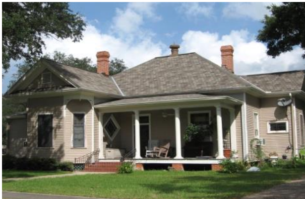
Tall, steep roofs like this one at 614 Adams Street were commonly used on late 19th and early 20th century houses.
