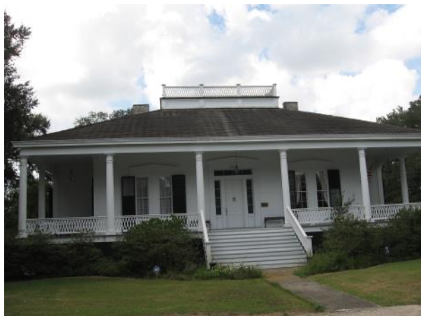
The Alfred Gates House at 205 Main Street retains many of its Greek Revival features like its porch columns and symmetrical plan.
