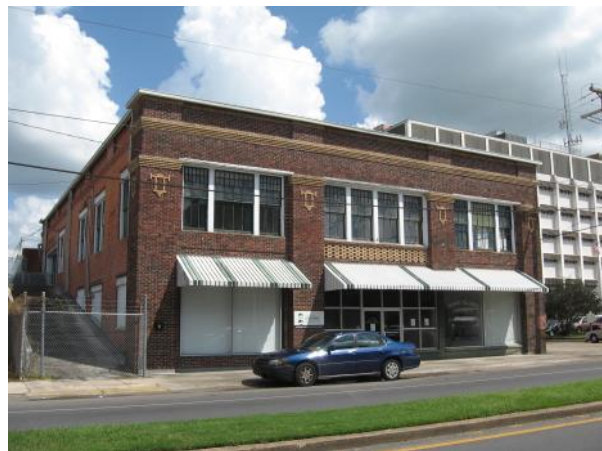
The building at 600 Main Street features typical elements of a two-part commercial building, including display windows on the first level, awnings over the windows, and double-hung sash windows on the second floor, and decorative brick design in the upper façade.
