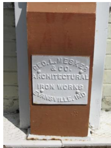
Cast iron name plates like the one on 700 Main Street were often found on commercial buildings from the late 1800s and identify the iron works manufacturer.
